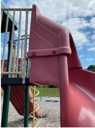
2022-11: Little Tikes Play Equipment missing hardware. Replace missing hardware.
